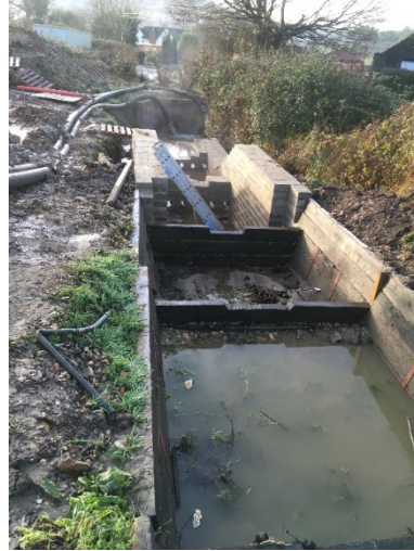
v. New check weir installations
