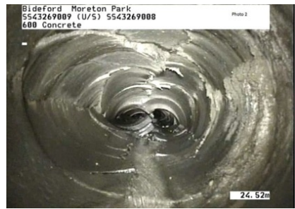
i. CCTV images showing collapsed culvert and a ground level image taken of the sinkhole.
