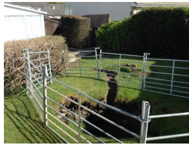
i. CCTV images showing collapsed culvert and a ground level image taken of the sinkhole.
