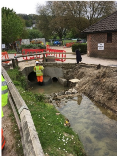
ii. New bypass culvert
