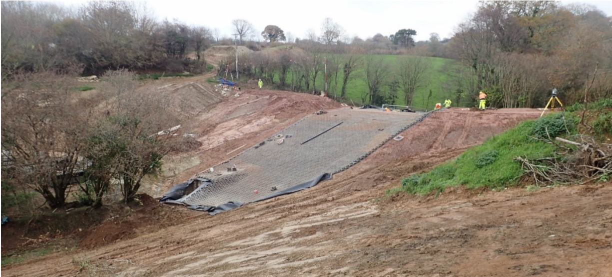
i. Looking eastwards towards Area 2 bund, with scour protection laid (to be covered with topsoil and seeded)
